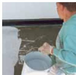
Naniesienie StoPur EB 200
